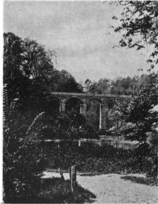
Railway Viaduct, near Midford.
